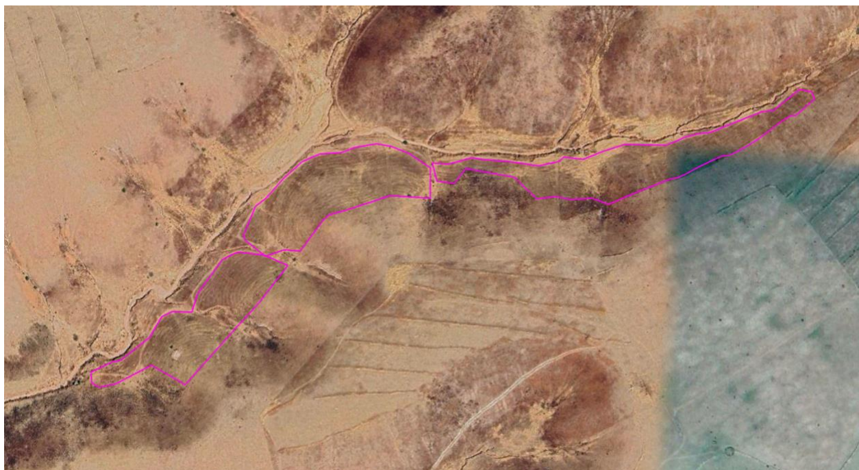
FIGURE 9. AERIAL PHOTO OF THE CONSTRUCTION SITE LAYOUT IN THE PROJECT AREA
